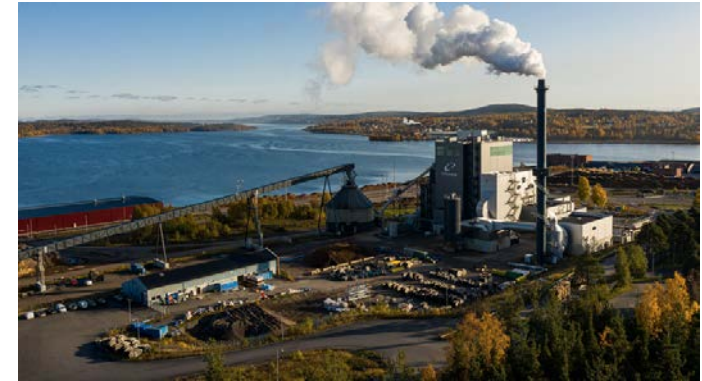
Sweden, Liquid Wind's production facility (@ Övik Energi)
