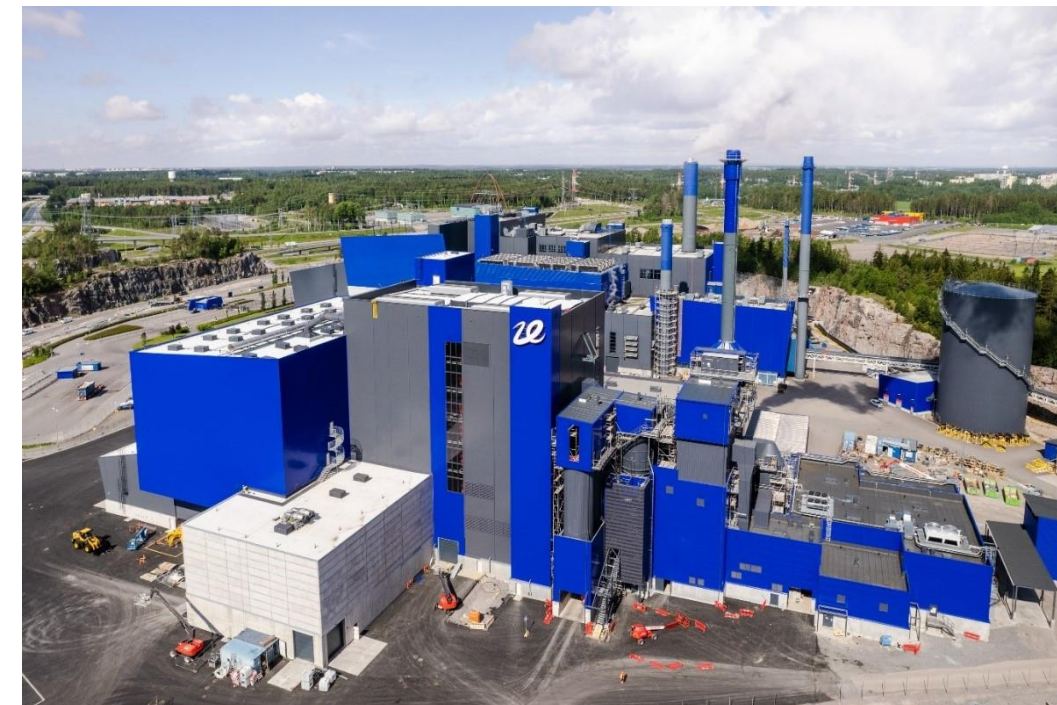
Vantaa Energy's Power-to-Gas integrated with Waste-to-Energy, Finland (Figure: Vantaa Energy)
