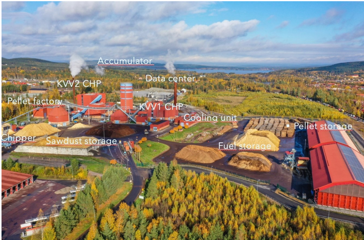
Figure 3: View of the plant Västermalmsverket in Falun. The two chimneys show the location of two parallel CHP units. The pellet plant is located to the left of these units, and a cooling plant to the right. In the center is the accumulator. Behind the plant (in grey) is the data center. We can also see storage of sawdust for the pellet plant, and different types of biomass for the CHPs: bark, woodchips, sawdust, recycled wood and discarded wood/fuelwood.
