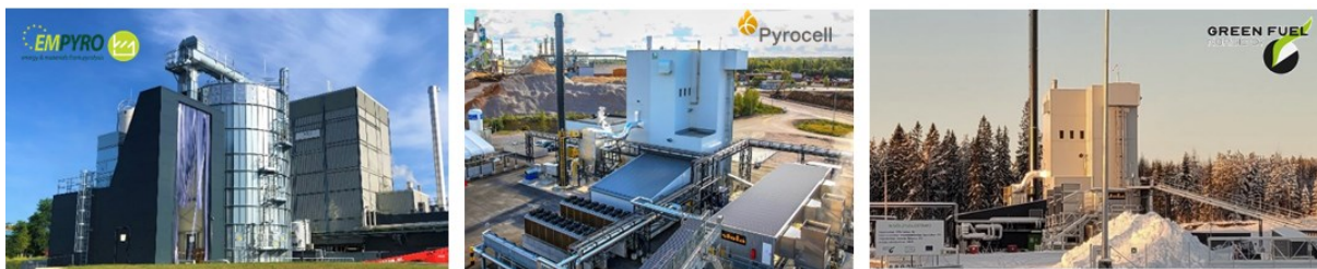
Fig. 2: Fast pyrolysis plants in the Netherlands, Sweden and Finland. Capacity 5 t/h biomass feedstock.
