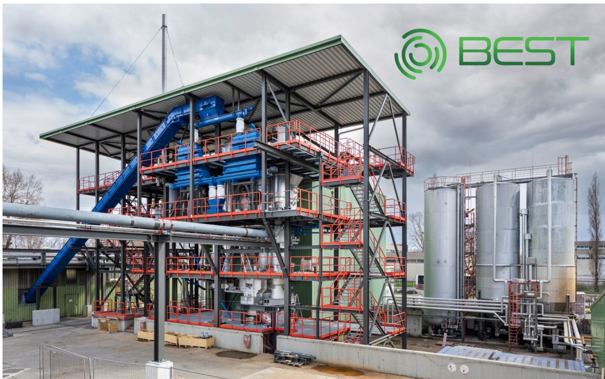
Figure 2: Photo of the dual fluidized bed (DFB) steam gasification process. The downstream synthesis is located in the green halls in the background. © BEST, 2021
