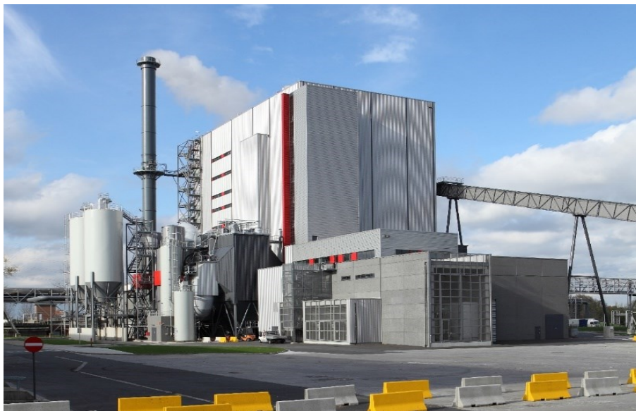
Figure 3: Stora Enso Langerbrugge utilizes renewable energy in paper production. Technology: Valmet CFB Boiler (circulating fluidized bed boiler) (source: Valmet Oyj)
